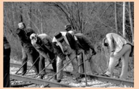
foreman typically positioned himself 50 yards or more from the section gang, squatted down, and examined the length of track for problems. He used visual signals to tell the caller where the track was out of alignment and when it was lined properly. At the time, rails typically came in 13-yard (12-metre) lengths. The section gang
